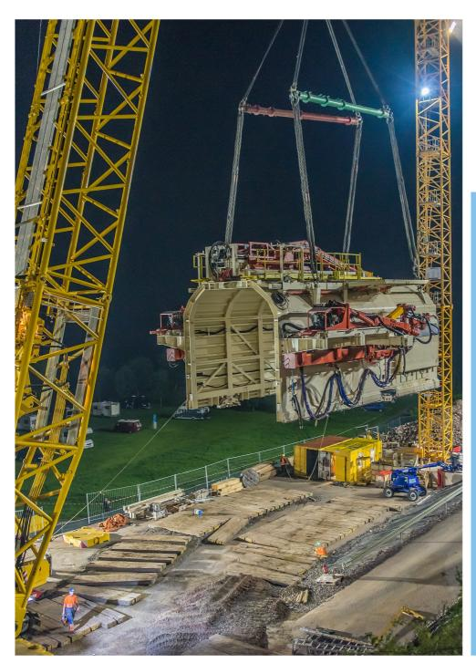
Railway tunnels have been in operation in Germany since the 19th century. The cross-section of these tunnels must be widened to meet the heightened safety requirements and speed increases. This also applies to the Petersberg Tunnel. In this case, a method is now being employed that has never been used before on an electrified line in Germany. Based on a protective gantry, the enlargement is being carried out during ongoing rail operations.
