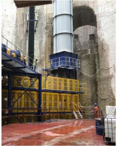
DS233 consists of five elements: a groundwater and storm water collection network, a drainage tunnel, which at 10.43 km is the longest in the region, a storage basin, a highly efficient pumping station and an outflow to the sea. The drainage tunnel will run from the Expo site, near the Sheikh Mohammed Bin Zayed Road and Jebal Ali Lehab Road to the sea and divert the rainwater and groundwater as a sewer system. Two CREG tunnel boring machines will take care of the tunnelling work.
